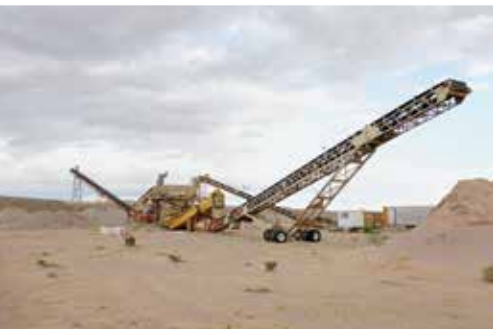
Complete Screen Plant | Las Vegas, NV, USA
