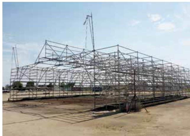
Large Quantity of Scaffolding | Tipton, CA, USA
